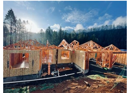
Rebuilding a Home Burned in the Holiday Farm Fire of 2020
